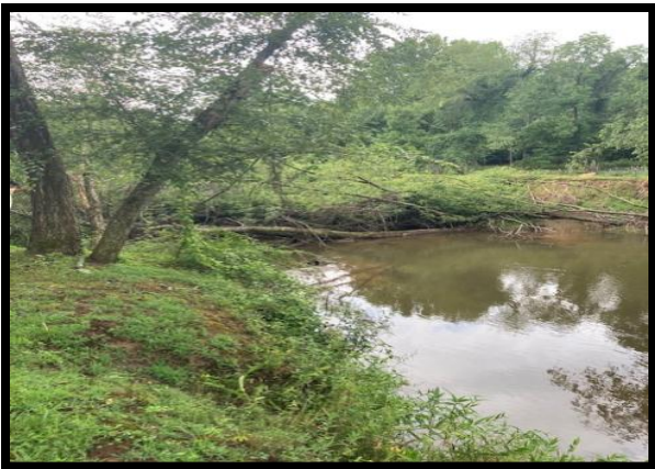
Brasstown Creek with severe blockages.
